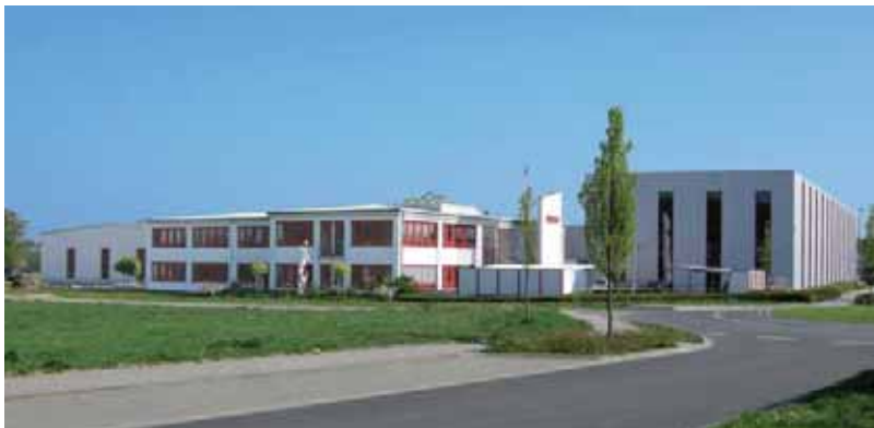
Hera headquarters in Enger
