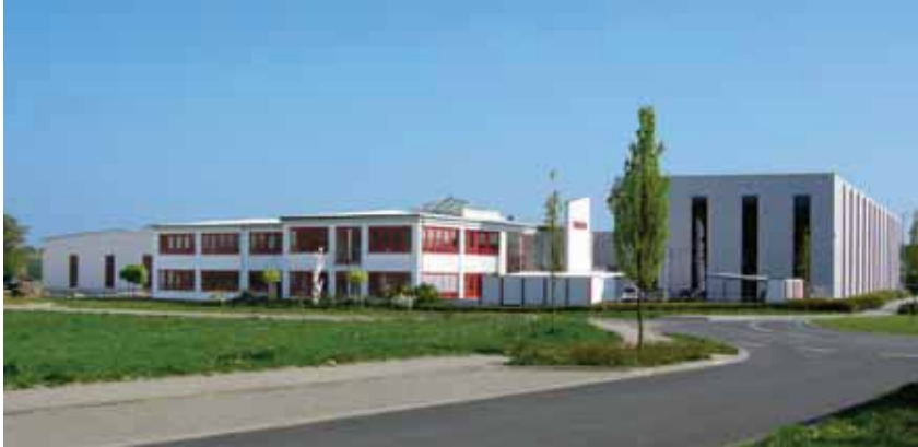
Hera headquarters in Enger
